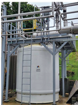
Figure 1. 10 kL helium dewar housing the 6 kW heater.
